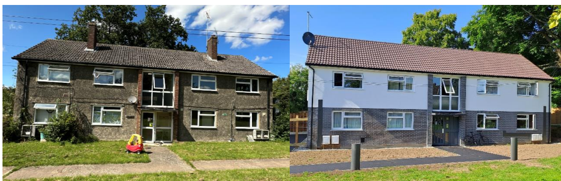
Figure 5. External appearance of Mount Pleasant properties before and after SHDF retrofits.
